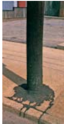
Creosote can migrate from treated poles causing contamination problems.
